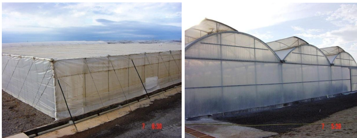
283 284 Figure 6: Examples of low-tech plastic greenhouse: the traditional low-cost ‘parral’ (left), which is widely used 285 in the Southern Spanish region of Almeria, and the more innovative pre-fabricated arch-shaped multi-tunnel 286 (photos: Alberto Pardossi)
